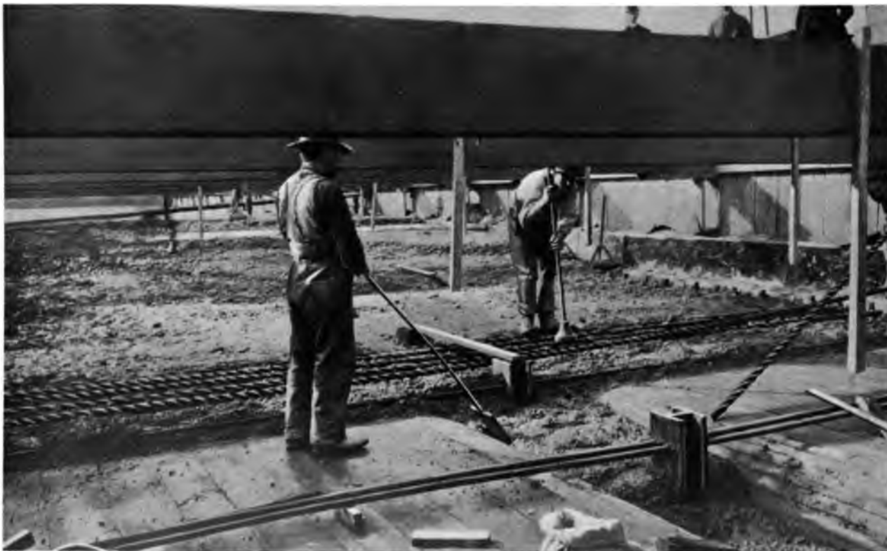
ROOF SHOWING CONCRETE-STEEL CONSTRUCTION — LENOX AVENUE AND 140TH-141ST STREETS
